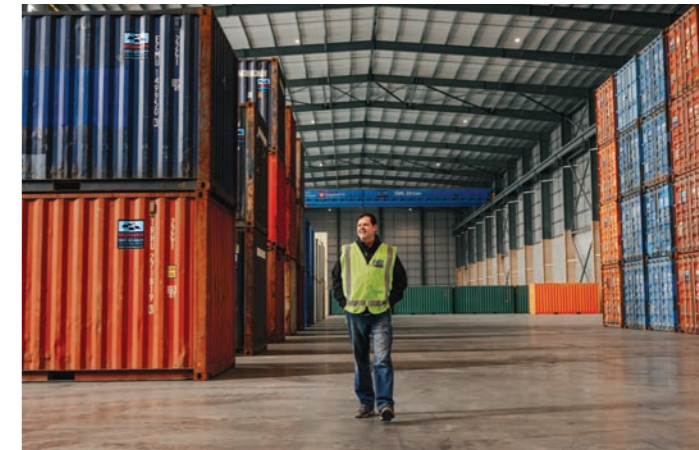
The Boxman building can store 2,600 shipping containers and deliver them to clients by automated gantry crane.
